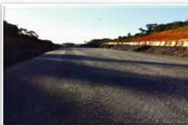
Preparation of sub base
