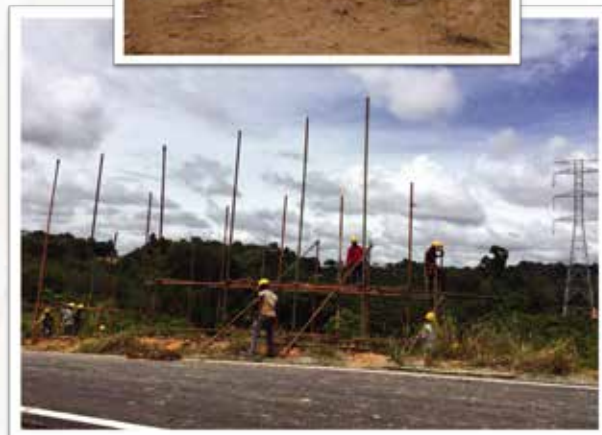
Scaffolding erection for road crossing at T5/5
