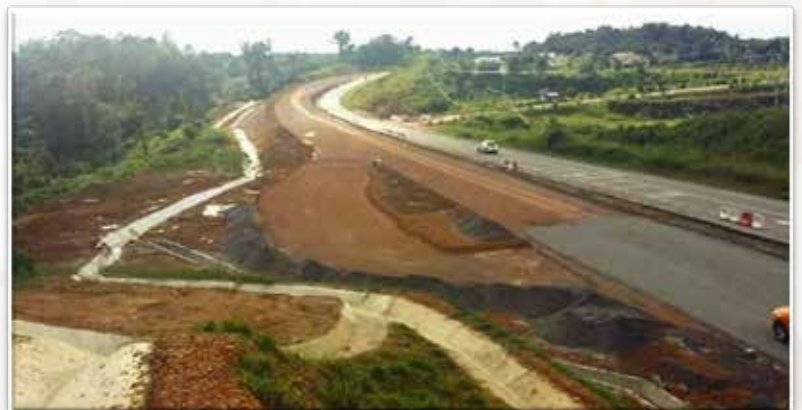
2nd Line road preparation
