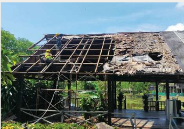
Repair works to existing timber structure in progress
