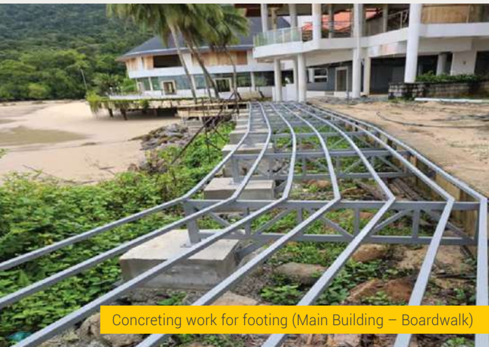
Mild Steel Installation Work (Ocean Wing)
