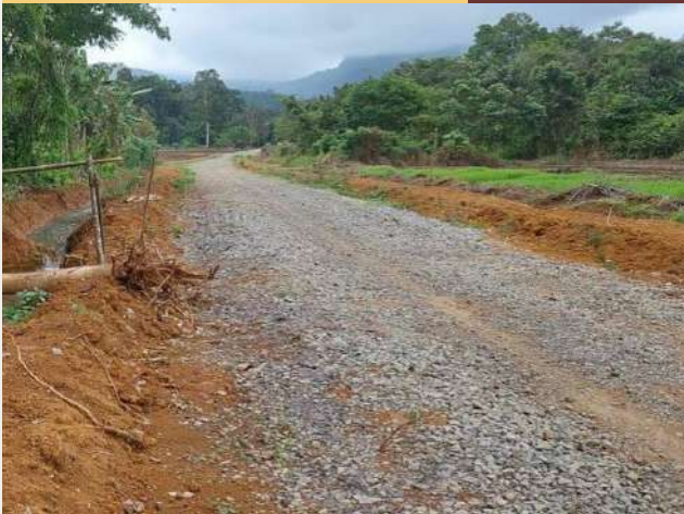
Before excavation work
