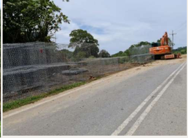
Remedial Works : Slope Failure
