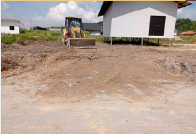
Road Base/Stoning Works
