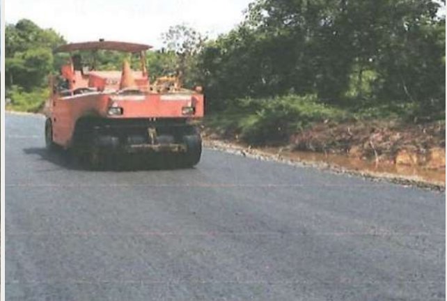
Ongoing road shoulder and roadline marking
