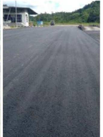
Completion of premix (ACW20)
