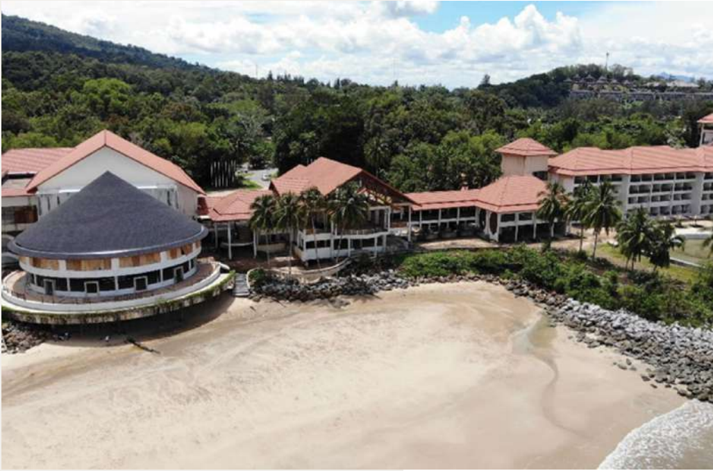
<<< DLR Phase 1 - Roofing Package Progress Spa Wing
