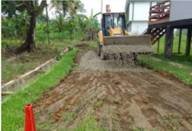
Road Base/Stoning Works
