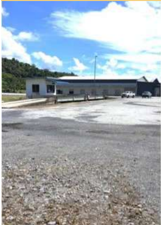
Platform for installation / construction of premix (ACW20)
