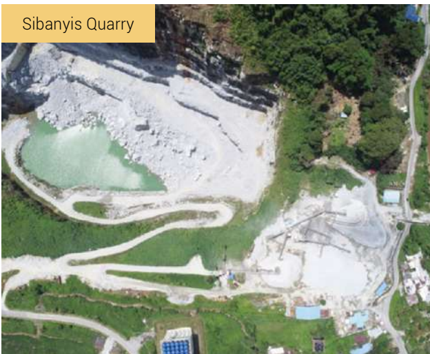
Conducted production optimisation exercise and added five units of heavy machinery .
