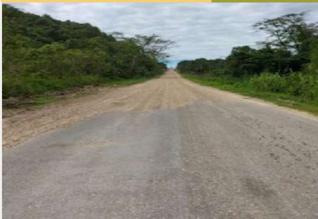
Remedial Works : Slope Failure
