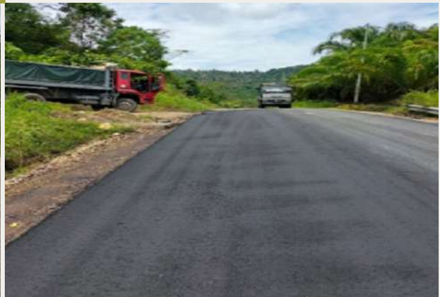
Remedial Works : Slope Failure
