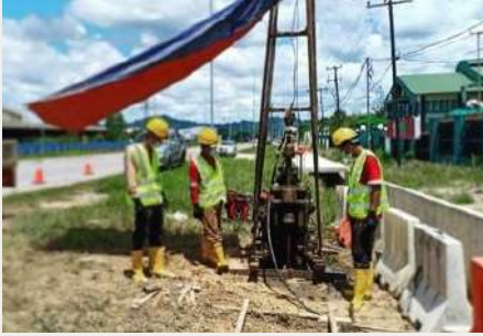
▲▲ The soil investigation work for the KUTS Project.
