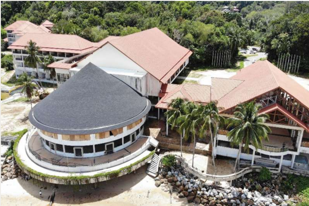
<<< DLR Phase 1 - Roofing Package Progress Baruk
