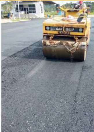
Installation / construction of premix (ACW20)
