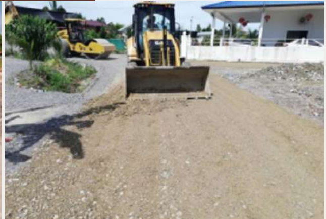
Road Base/Stoning Works
