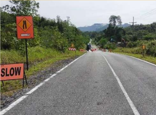
Excavation Work In Progress
