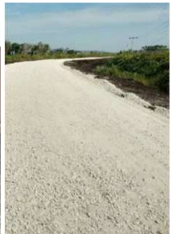
Completion of stoning
