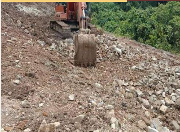
Excavation Work In Progress
