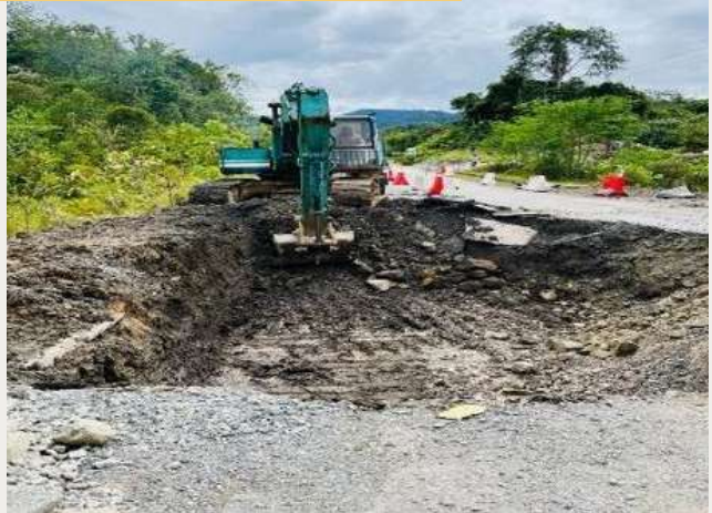
Excavation Work In Progress
