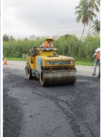
Laying of Premix
