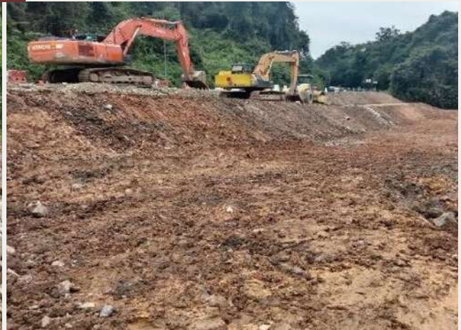
Excavation Work In Progress
