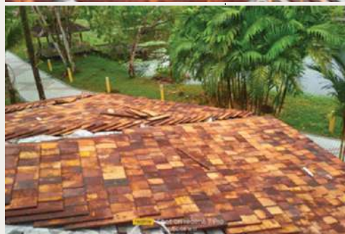
<<< Installation of belian shingle in progress
