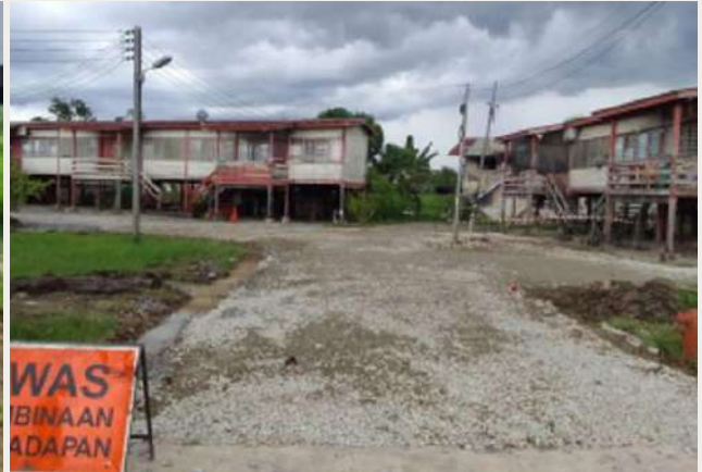
Road Base/Stoning Works
