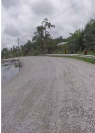
Laying of Stoning
