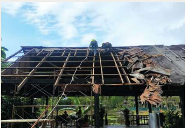
Dismantling works of existing roof material
