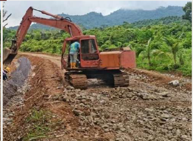
Excavation work in progress
