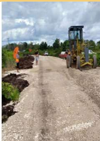
Installation / construction of stoning
