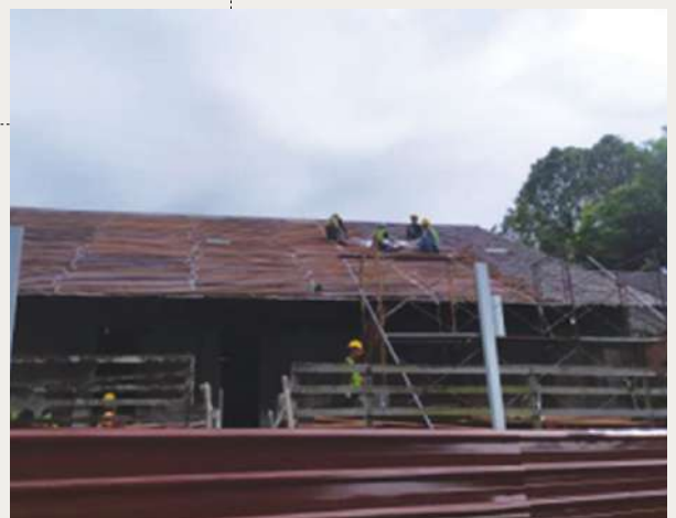
>>> Installation of GI sheet in progress
