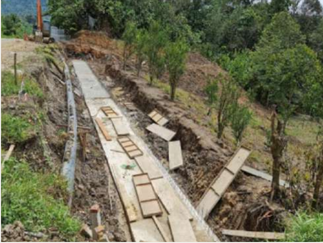
Remedial Works : Slope Failure
