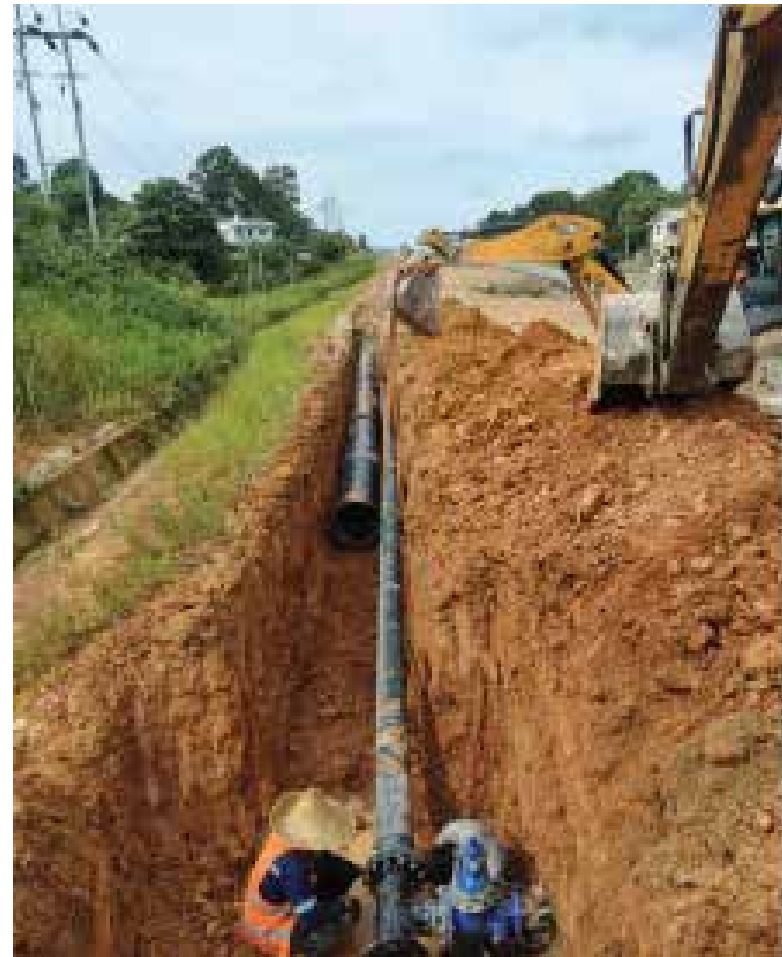
Pipe laying works carried out by the site team
