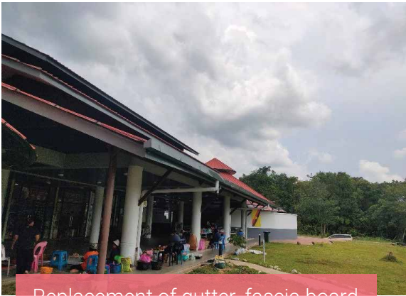
Replacement of gutter, fascia board and downpipe completed
