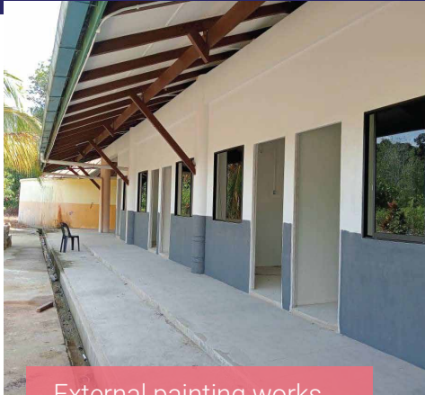
External painting works
