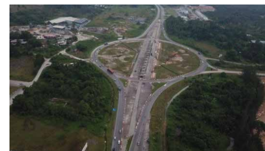
Aerial view of a section of the KUTS Project's Blue Line along the Kuching-Samarahan Expressway in Kota Samarahan, which served as the 3km test route for the ART Proof-of-Concept (POC) exercise.
