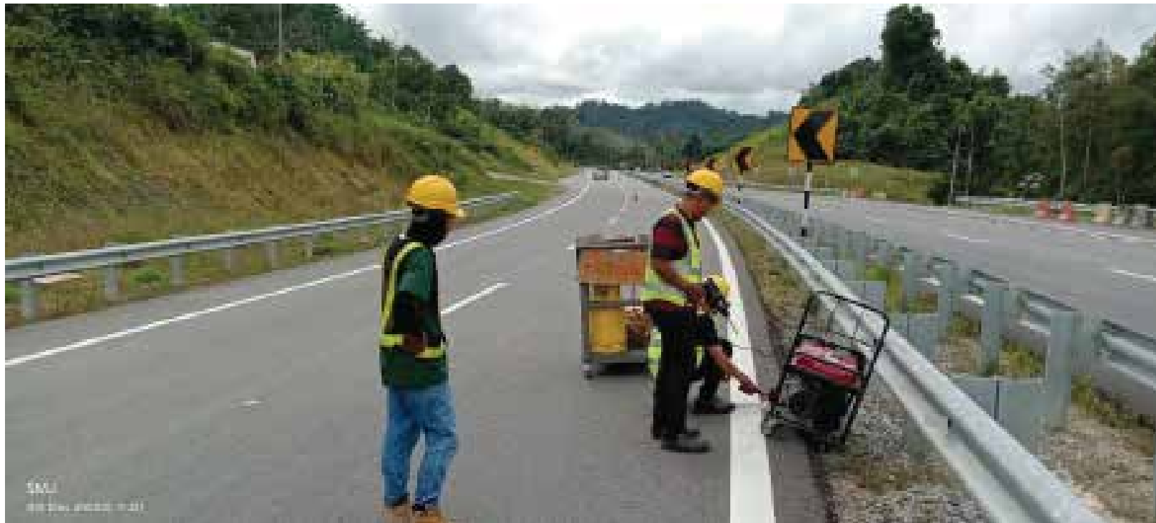
Road stud marking works
