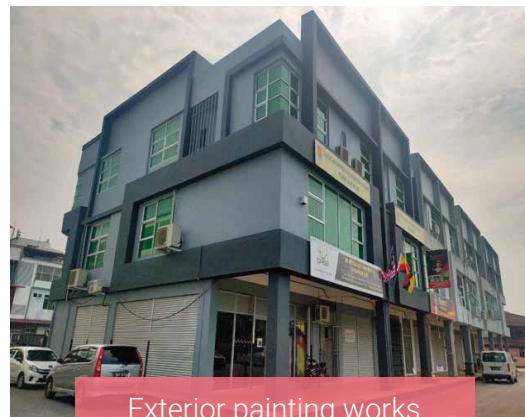
Exterior painting works
