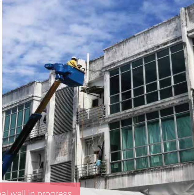
Cleaning of external wall in progress
