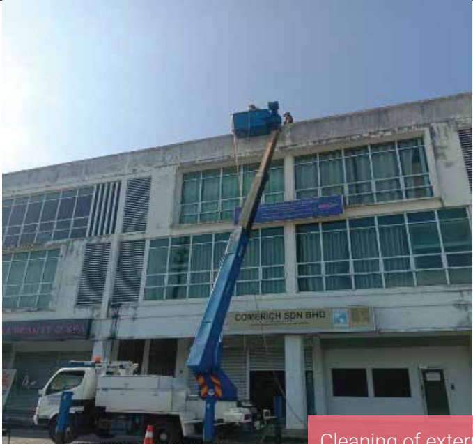
Cleaning of external wall in progress
