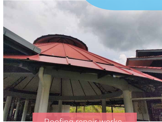
Roofing repair works
