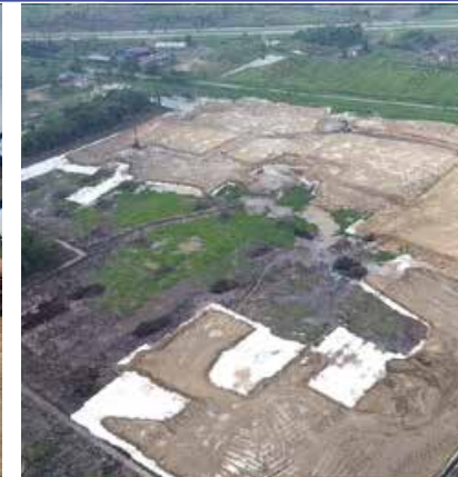
Aerial view of Rembus Depot construction site
